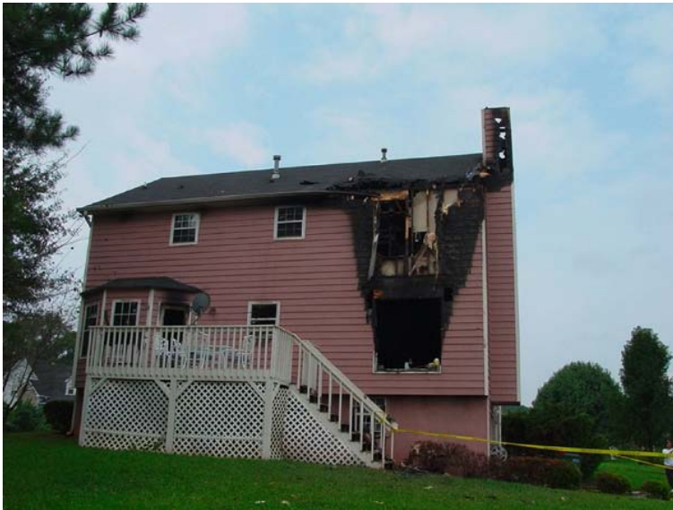
FIGURE 18.2 The gaping hole in this house was caused by lightning. When it struck the house, it caused a major fire and extensive damage. Such direct hits on buildings, especially those with lightning rods, are relatively rare. Courtesy: John Lentini
