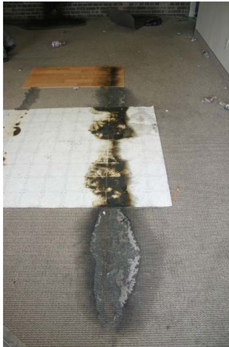
FIGURE 18.6 A fire trail made by pouring a flammable liquid on a floor. Note the irregular pattern of burning caused by pouring the liquid out of some container such as a bucket.
