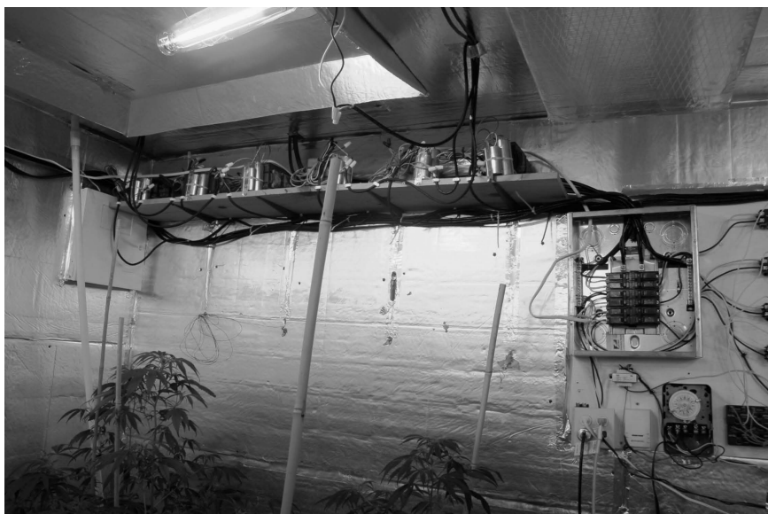
Figure 8.2 Transformers to distribute power.
