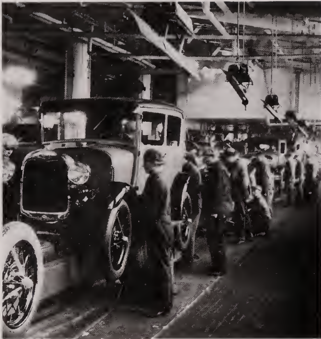
The ideas of scientific management were most successfully applied by Henry Ford, who pioneered the automobile assembly line. As shown in this 1928 photograph of the Dearborn, Michigan, plant, Ford divided up the job of building cars into hundreds of different tasks, each performed by a worker as the cars moved along an assembly line. The result was that new cars could be produced so cheaply that most of these autoworkers could afford to buy one.
