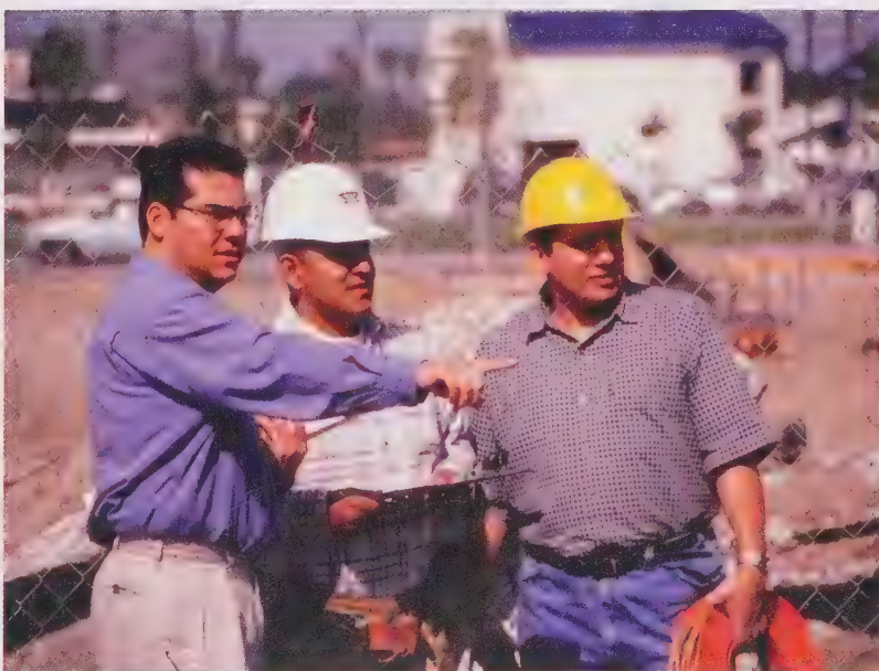
On a construction site
